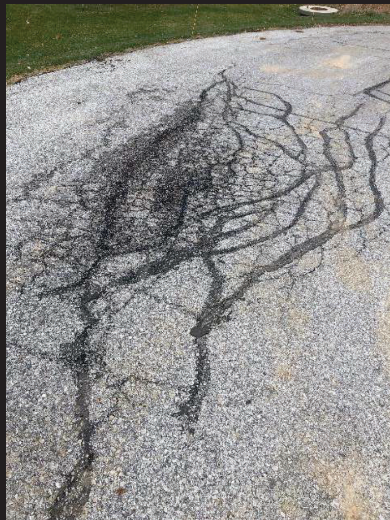
Moisture Invasion & Wheel Pressure related Damage
