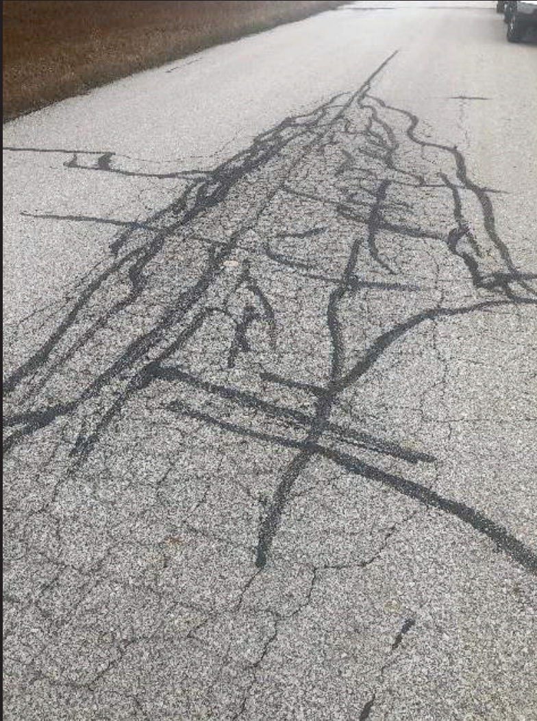
Current Raveled Surface in Area #7
