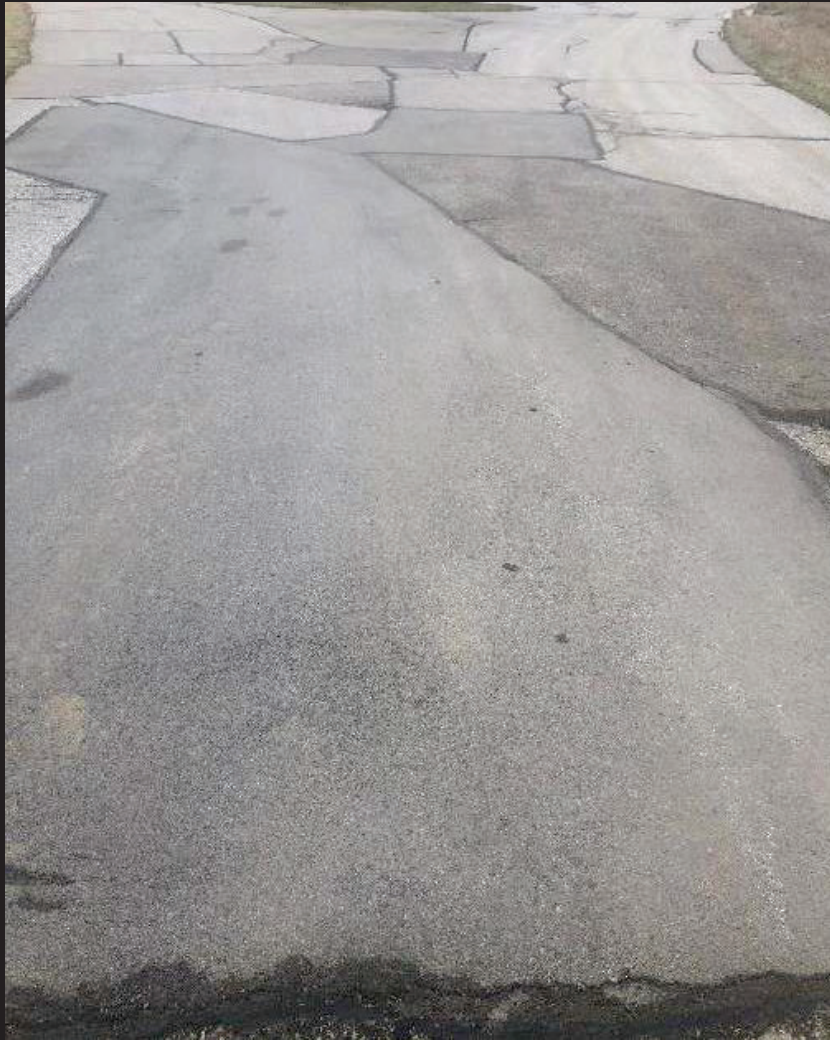
Multiple Patches in Area #1 – Further Moisture Damage Eminent
